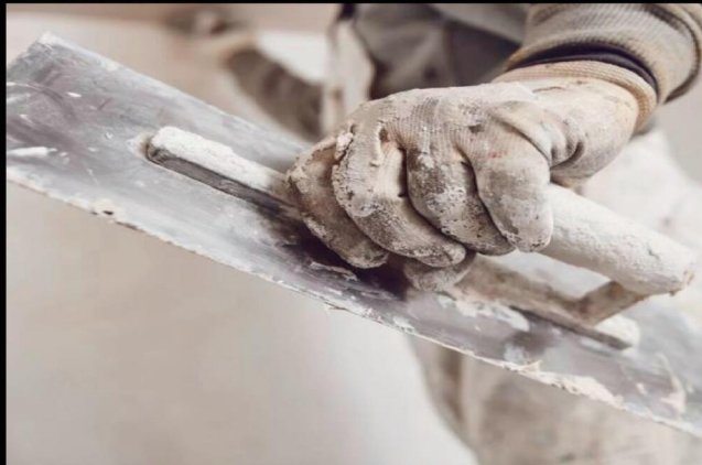
GARAGE CONVERSIONS PLASTERING
