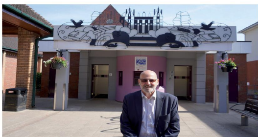
Phil Childs, Wychavon's street scene and amenities officer, in front of the revamped St Andrews Square toilets in Droitwich. s
