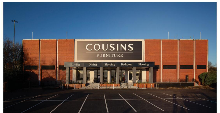
New modern entrance at Dudley store completed 2024.
