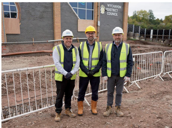
Speller Metcalfe contracts manager, Richard Monk, Wychavon Leisure's managing director, Nigel Grundy, and Speller Metcalfe's project manager, Sean McDermott, at the site. Picture by Wychavon District Council.
