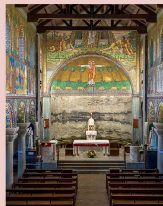
The mosaics are looking magnificent after their refurbishment.
