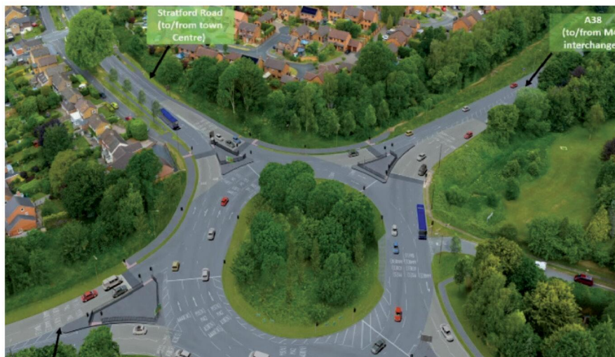
How the new-look Oakalls Island will look when work is completed. Picture by Worcestershire County Council. s
