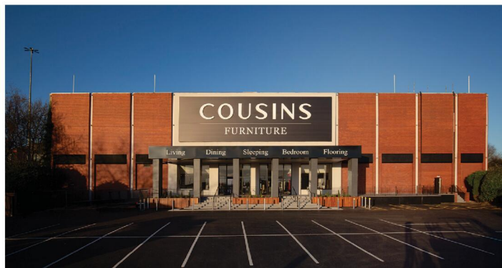
New modern entrance at Dudley store completed 2024.
