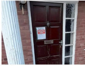
The houses were issued with emergency closure notices. s
